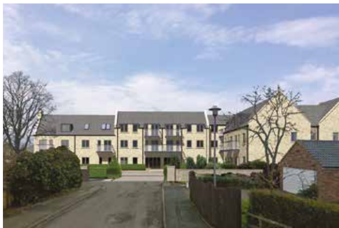
Start on site for Box Tree Court (Boston Spa)
