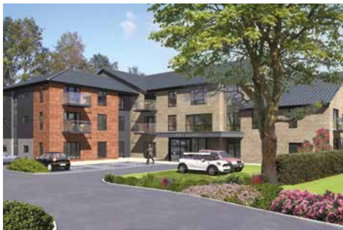
Start on site for Fry Court (Great Ayton)
