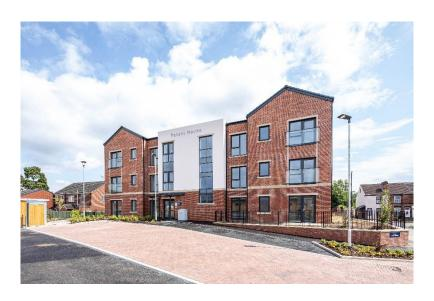
Our pioneering Patent House and Patent Walk scheme is England's largest net-zero Retirement Living complex to be built using volumetric modular construction — where large, enclosed, pre-made and fitted out sections are joined together on site to form a complete building.
